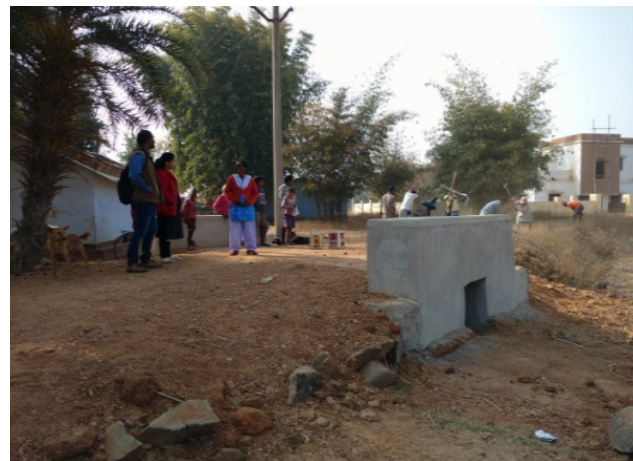
RCC Bridge being constructed in Panchayat
