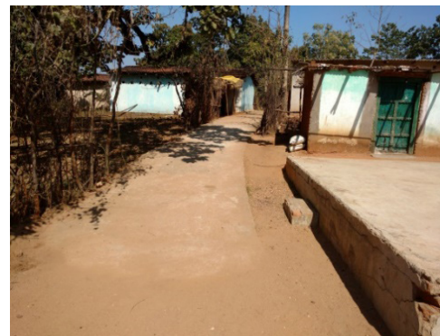
Road constructed in Ichak Gram Panchayat
