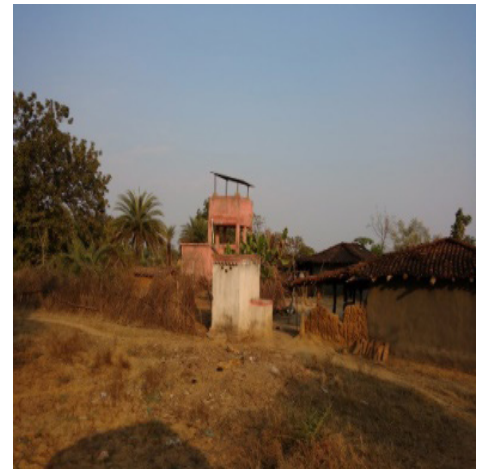
Community water tank constructed during first tenure of Ashren Kerketta
