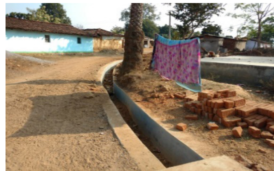
A drainage system constructed in Karenjoba Gram Panchayat
